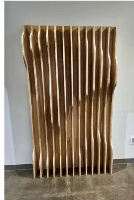
Wall slat system with plywood back panel – no visible hardware
