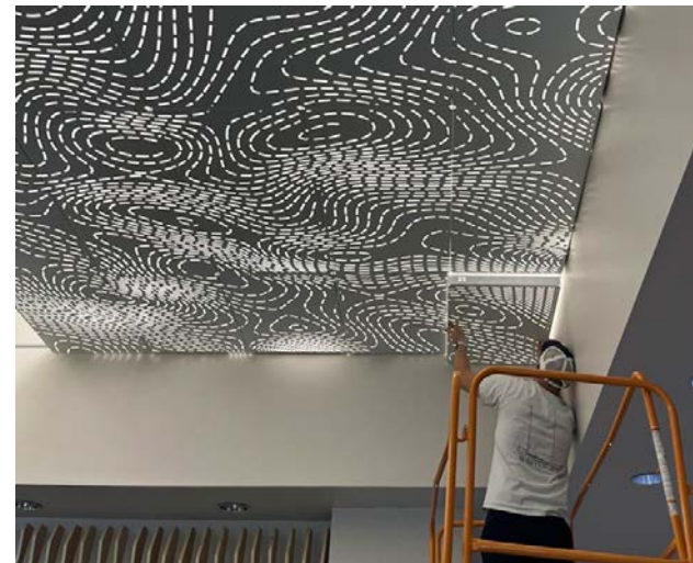
All tiles are numbered with the associated final schematic to ensure ease-of-installation
